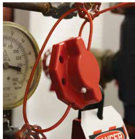
Turn the hasp halves to cinch cable.
