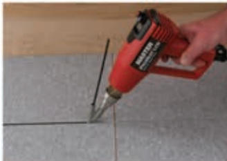
Welding Flooring Material
