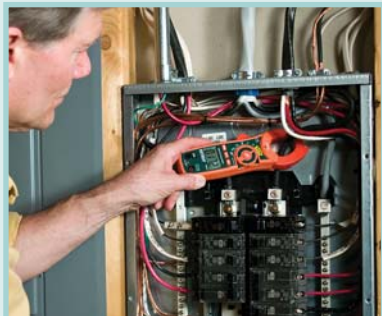
Compact size allows measurements in tight locations
