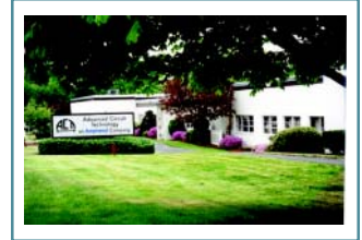
Amphenol Advanced Circuit Technology facility in Nashua, NH houses the manufacture, design and engineering of flex circuit products.
