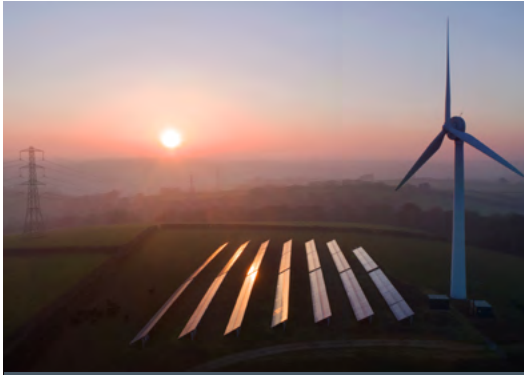
Energy and power
