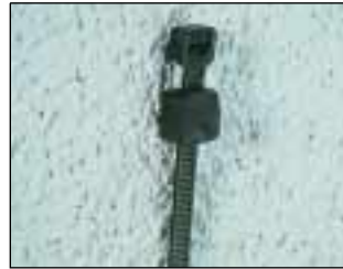
3. Place cable tie through mount.
