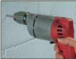
1. Drill hole using correct size bit.
