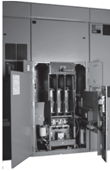
50L7 Vacuum Retrofit
