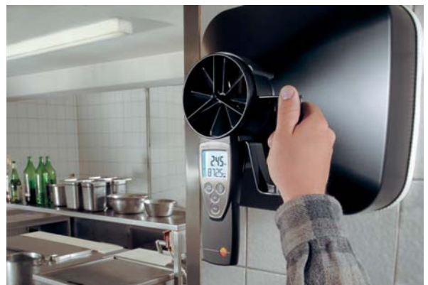
Using the testo 417 to monitor the exhaust air at a wall-mounted ventilator
