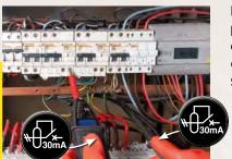
By simultaneously pressing the double command, you can cause a fault current sufficient to trip the RCD to flow through a low-impedance load.
